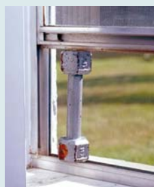
Window balances broken
